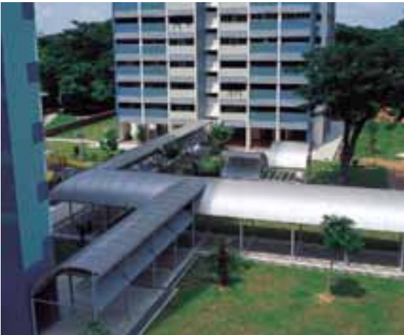
Roof of pedestrian passage, Singapore
