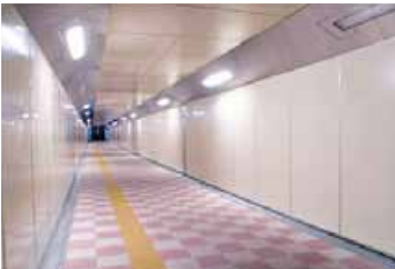
Pedestrian underpass lining, Japan
