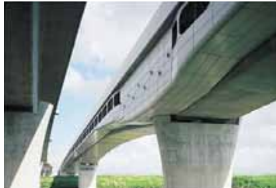
Cable cover of bridge, Japan
